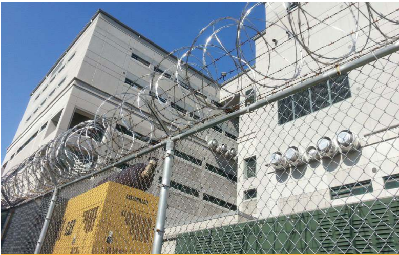
Etowah County Detention Center in Gadsden, Alabama
