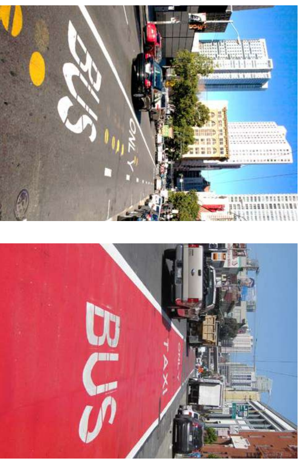
FIGURE 11 SAN FRANCISCO 3RD STREET TRANSIT-ONLY LANE BEFORE AND AFTER RED TREATMENT AND CORRESPONDING VIOLATIONS PER HOUR ALONG THE CORRIDOR
