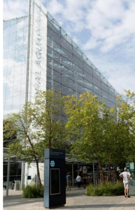
National Aquarium “wing wall”. Design credit: Ayers Saint Gross
