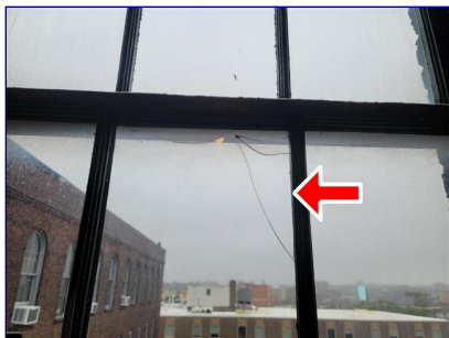
1.5 Item 1(Picture) bathroom
