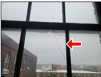
1.5 Item 1(Picture) bathroom
