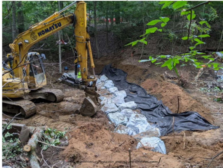
Camp Woodlands Stream Restoration (Broad Creek), Anne Arundel Co.
