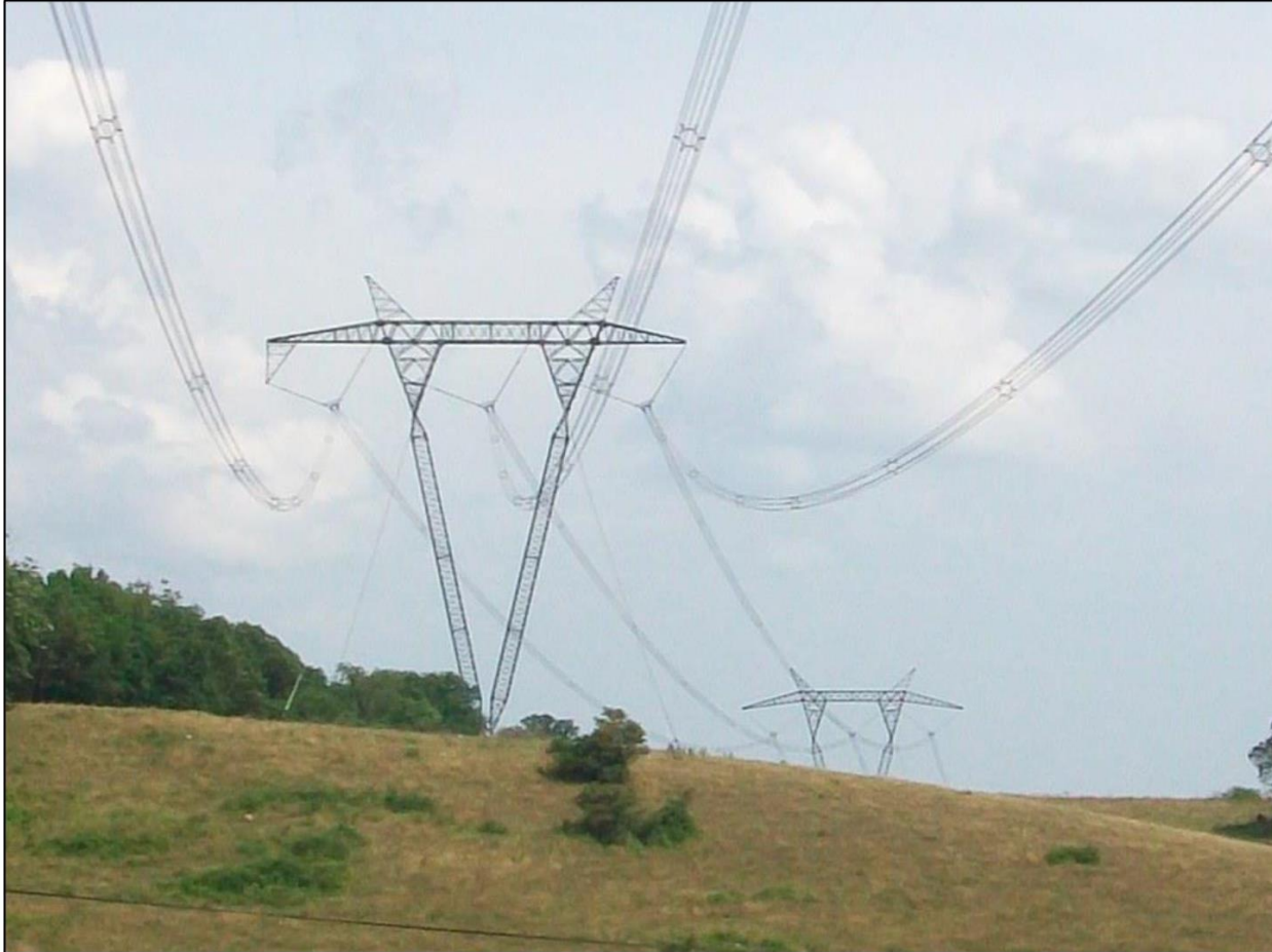
765kV Guyed-V Lattice tower
