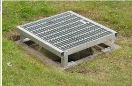
Raised Grate Yard Inlet
