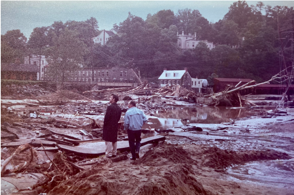
Hurricane Agnes (1972) Destruction along the Patapsco River in Baltimore County.
