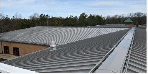
A standing seam metal roof replaced a 52,000sf asphalt shingle roof at Green Holly Elementary School in St. Mary's County.
