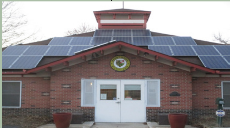
Brentwood Solar Panels on Town Hall
