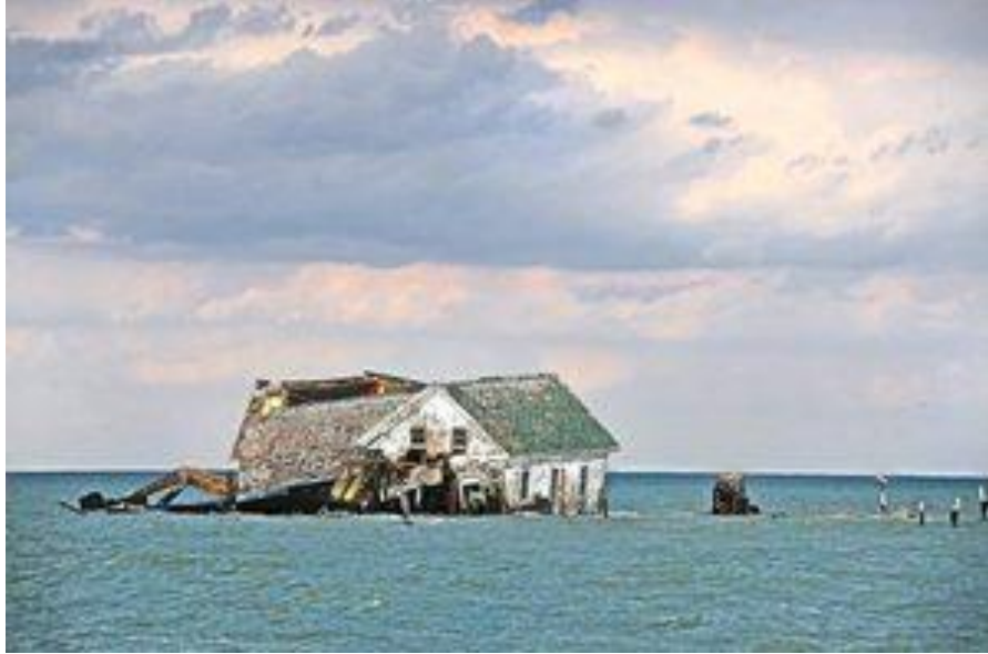
Last House on Holland Island Collapses; Photo from The Seattle Times
