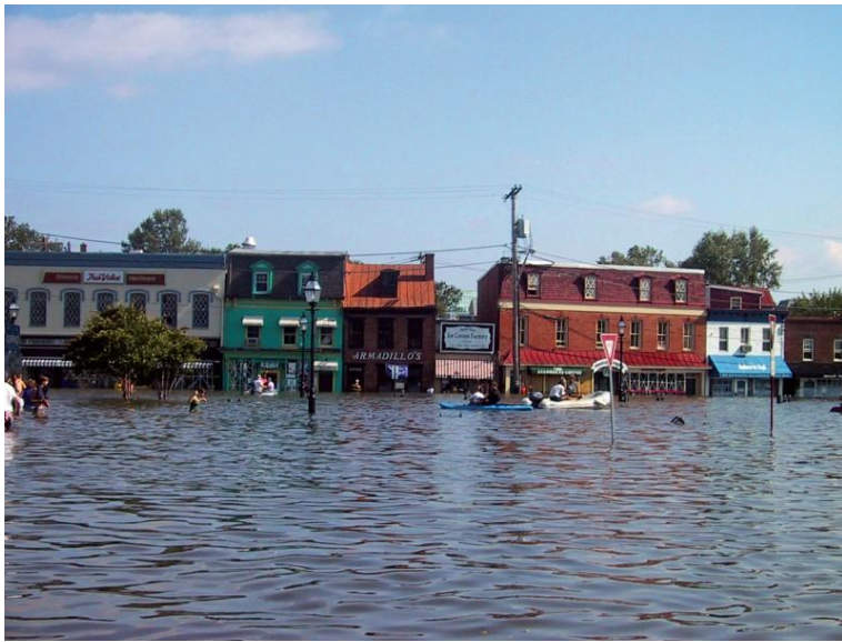
Flooded Downtown Annapolis; Photo from the State of Maryland
