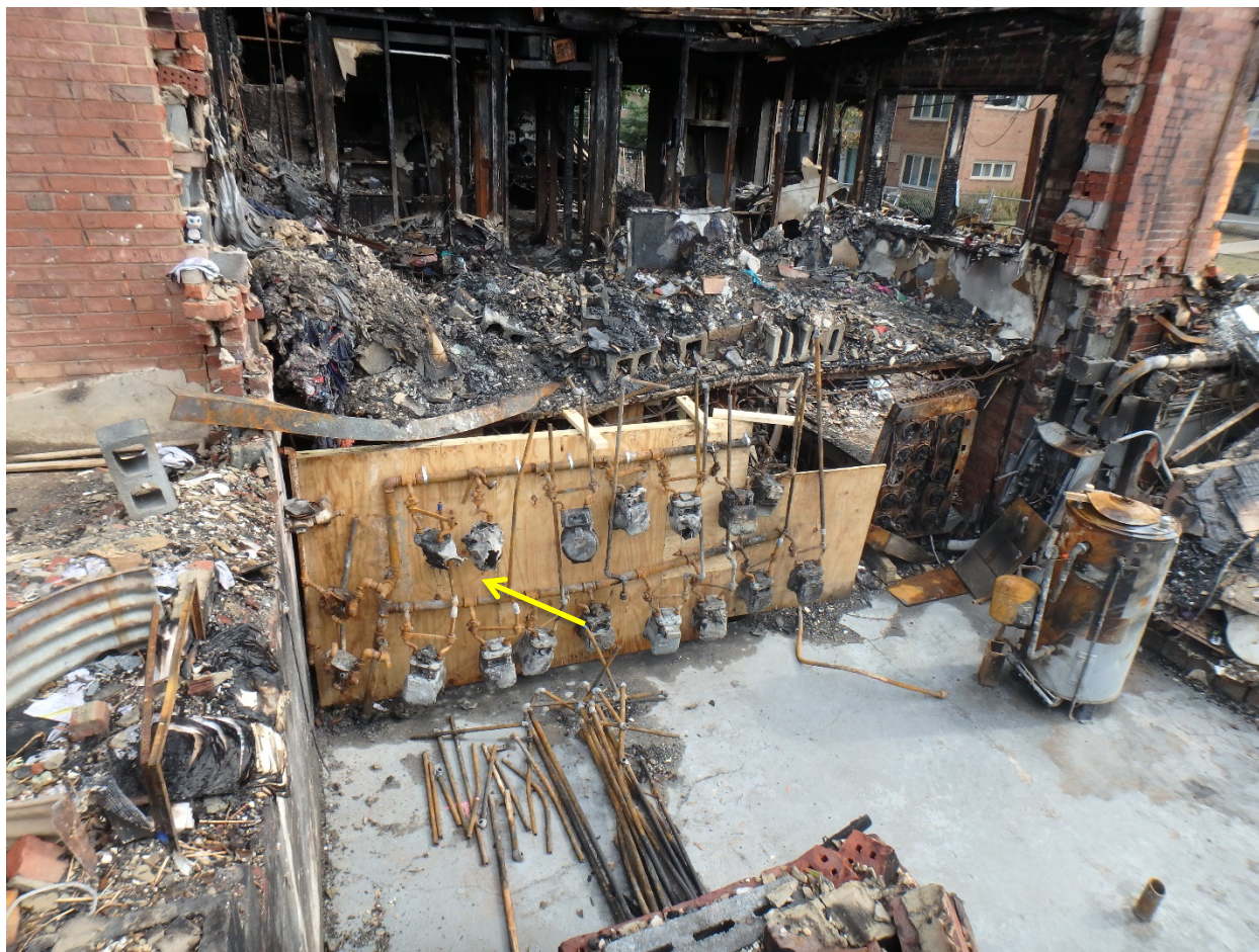
Figure 6. Building 8701 after debris removal and ATF reconstruction. The first two gas meters (designated with a yellow arrow) show substantially more heat/fire damage than other meters. (Photograph provided by ATF.)
