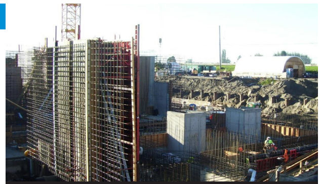
Anacortes, WA Water Treatment Plant Watertight Construction
