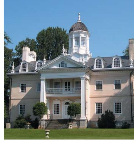
Figure 37: Current lawn entrance view of Hampton
