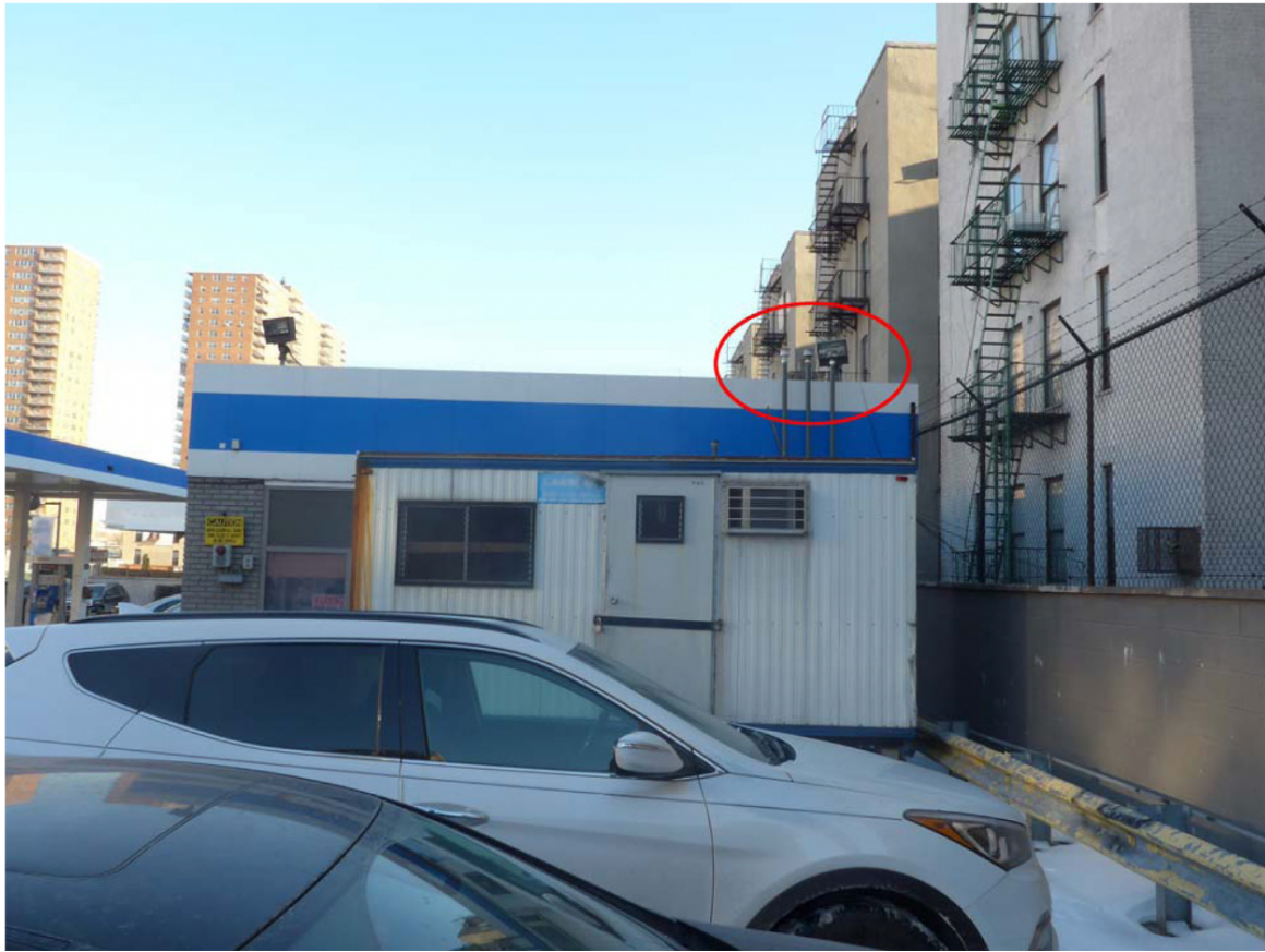
Figure 3: The three vent pipes (enclosed by the red ellipse) on the right side of the convenience store of a gas station are less than 10 m away from the residential building. Source: Hilpert et al. (2019).
