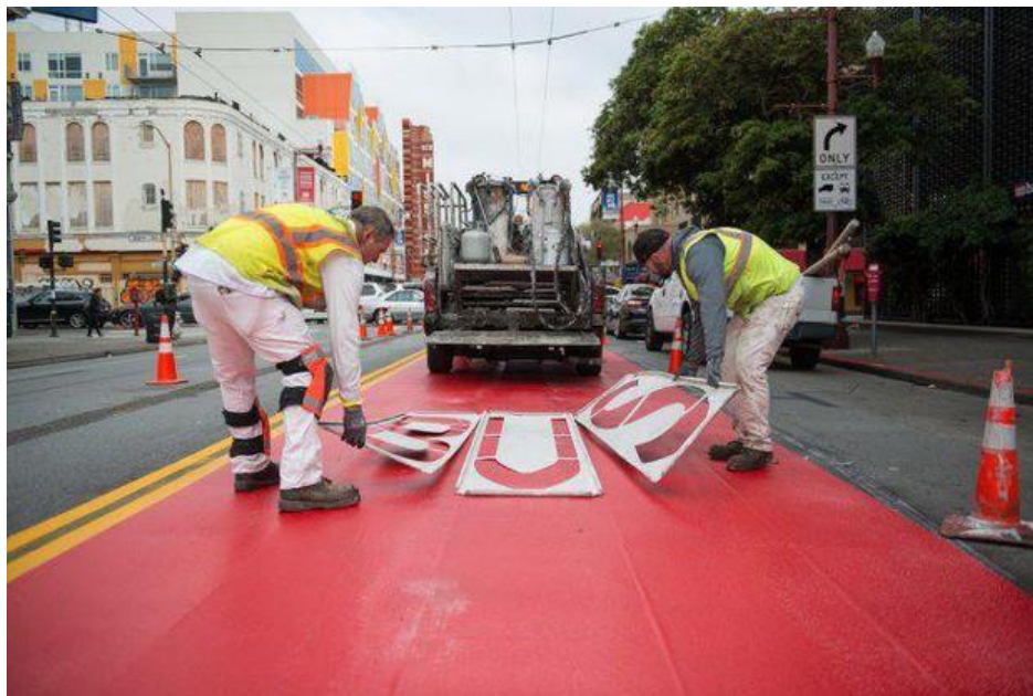
Workers make a bus lane permanent in San Francisco. (SFMTA)
