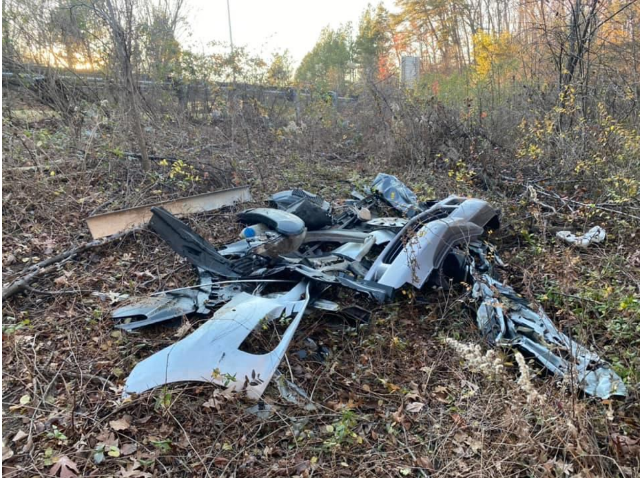
I-195 @ MD 295 (Anne Arundel Co.): The remains of SIX different vehicles were found in one spot where a recent guardrail repair was done. Pieces of the guardrail were also tossed behind the repaired guardrail after all these materials were brought to the shoulder for removal.
