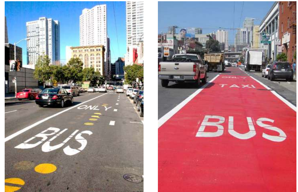
FIGURE 11 SAN FRANCISCO 3RD STREET TRANSIT-ONLY LANE BEFORE AND AFTER RED TREATMENT AND CORRESPONDING VIOLATIONS PER HOUR ALONG THE CORRIDOR
