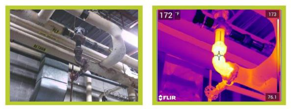
A Mechanical Insulation Energy Audit was performed, and it was determined that these 3 feet of missing insulation is costing the owner \$799.74 a year. The pipe repair was conducted 5 years prior. Without the insulation being replaced, it has costed a total \$3998.70 of energy loss. If the insulation was properly repaired costing \$500, it would have saved the owner \$3,498.70 in that same 5-year time period.
