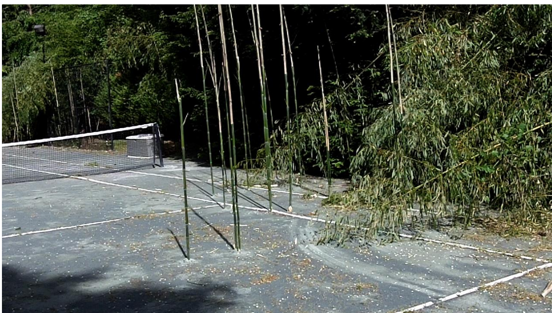
Stalks of invasive running bamboo coming up from underneath tennis court surface from rhizomes spreading underground from bamboo grove
