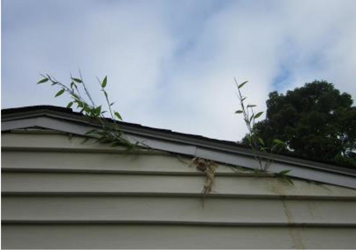
Running bamboo leaves emerging from behind sheathing and siding
