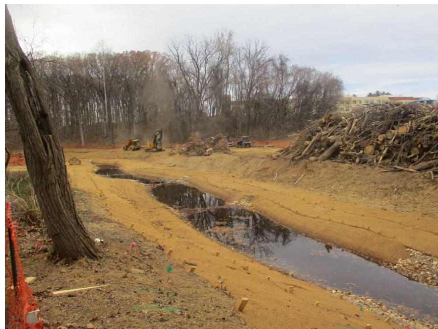
(Above: Solitaire Court stream restoration in Gaithersburg; photo by R. Portonova, 12/3/2021)
