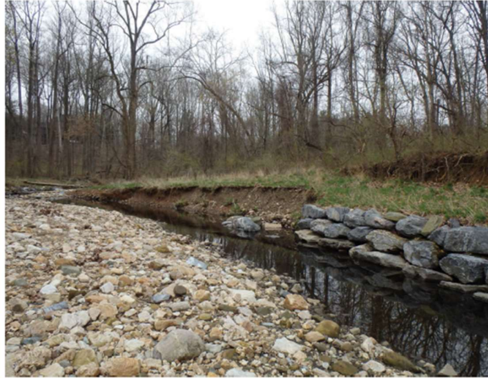
Lower Booze Creek - Erosion downstream of imbricated wall structure from original stream restoration.
