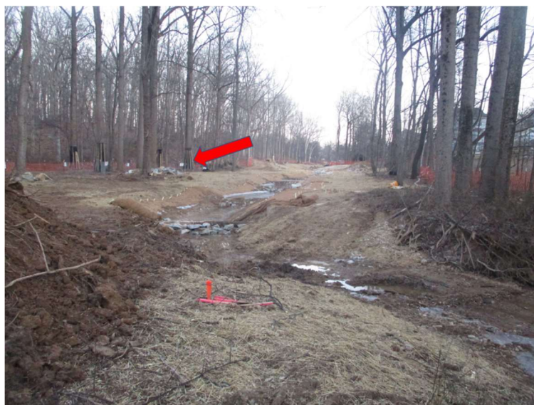
(Above: Solitaire Court stream restoration in Gaithersburg; photo by R. Portanova, 2/7/2022)
