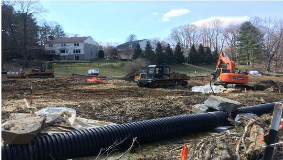
(Above: Falls Reach Stream Restoration Project; photo by K. Bawer, 3/19/2019)
