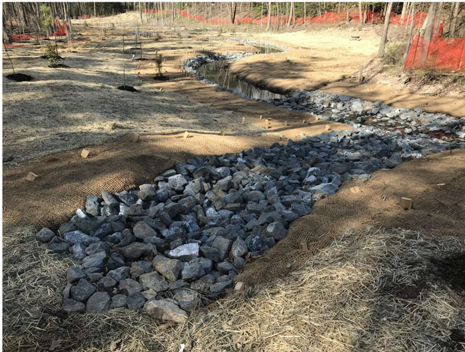
(Above, St. Charles Parkway stream restoration, Charles County; from https://www.charlescountymd.gov/our-county/infrastructure-capital-services/npdes-project/st-charles-parkway#ad-image-0 )
