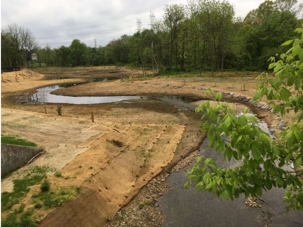
(Above: after construction: Whetstone Run in Blohm Park, Gaithersburg; by K. Bawer on 5/03/2021)
