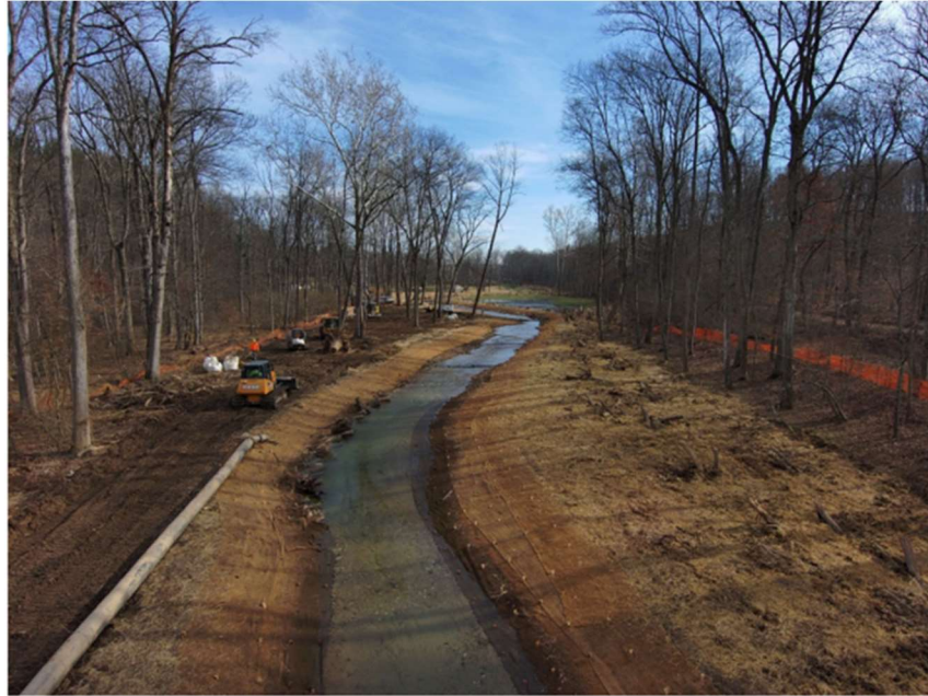
(Above: Mayberry Stream Restoration in Carroll County ; from https://www.carrollcountymd.gov/media/16472/mayberry-stream-restoration.pdf )
