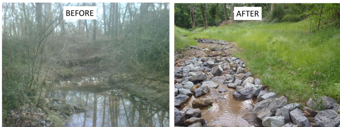
(From DPW, City of Takoma Park)
