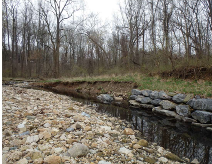
Lower Booze Creek - Erosion downstream of imbricated wall structure from original stream restoration.
