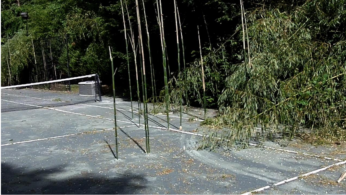
Stalks coming up through a tennis court pavement because rhizomes spread underground from the grove of invasive running bamboo
