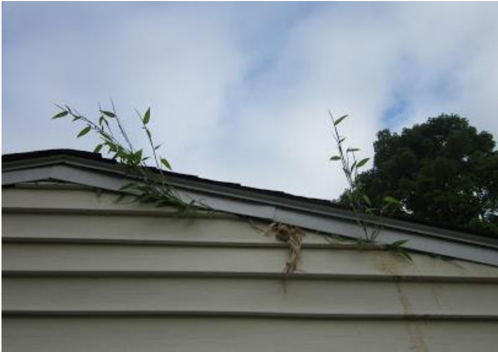
Running bamboo stalks and leaves emerging from behind the sheathing and siding
