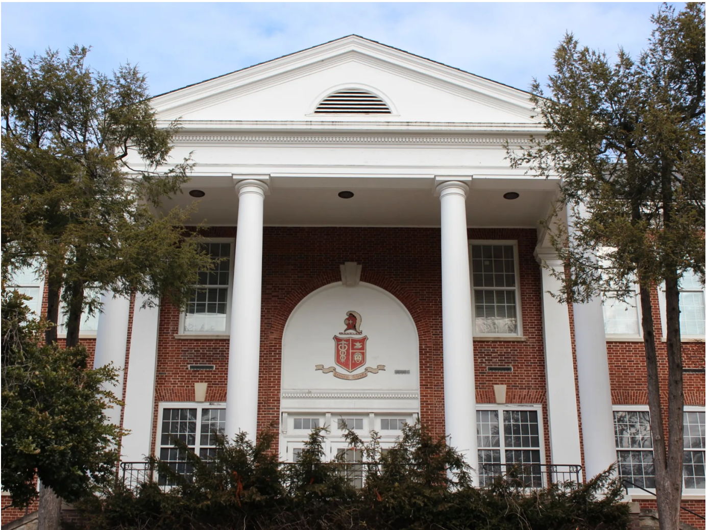
Exterior of Silver Spring International Middle School, which looks out over Purple Line construction on Wayne Avenue. Credit: Em Espey
