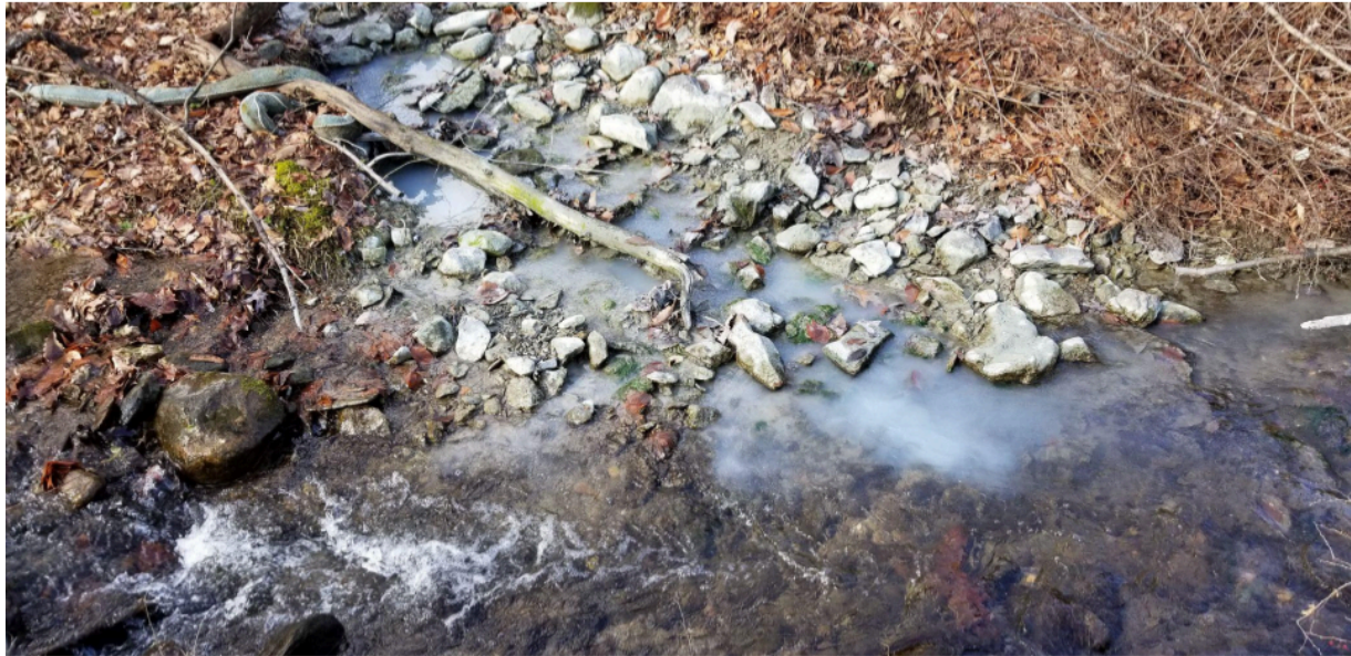
This photo is of the permitted discharge outlet from the stormwater pond. You can see the milky white pollution entering the stream.
