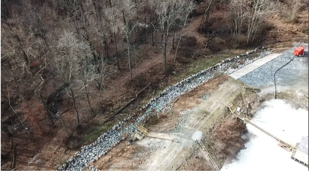
This photo shows the permitted discharge to Miney Branch. The Rock path is supposed to allow for solids to settle out before entering the receiving stream.
