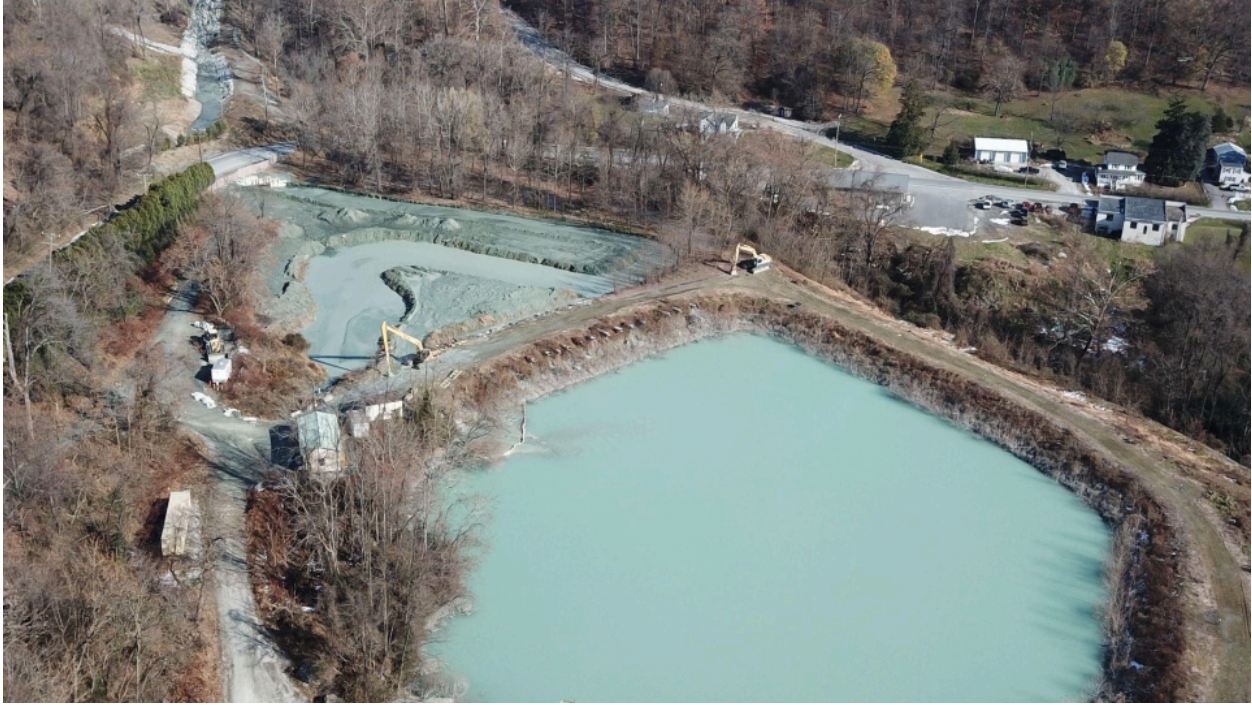
This photo shows a close up of the stormwater pond.
