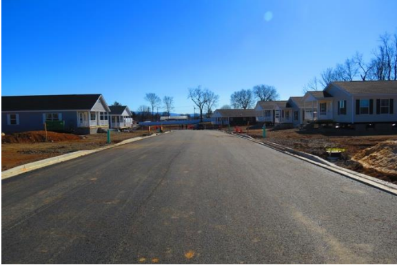
Streetscape: 1347-1367 Connecticut Ave Hagerstown, MD
