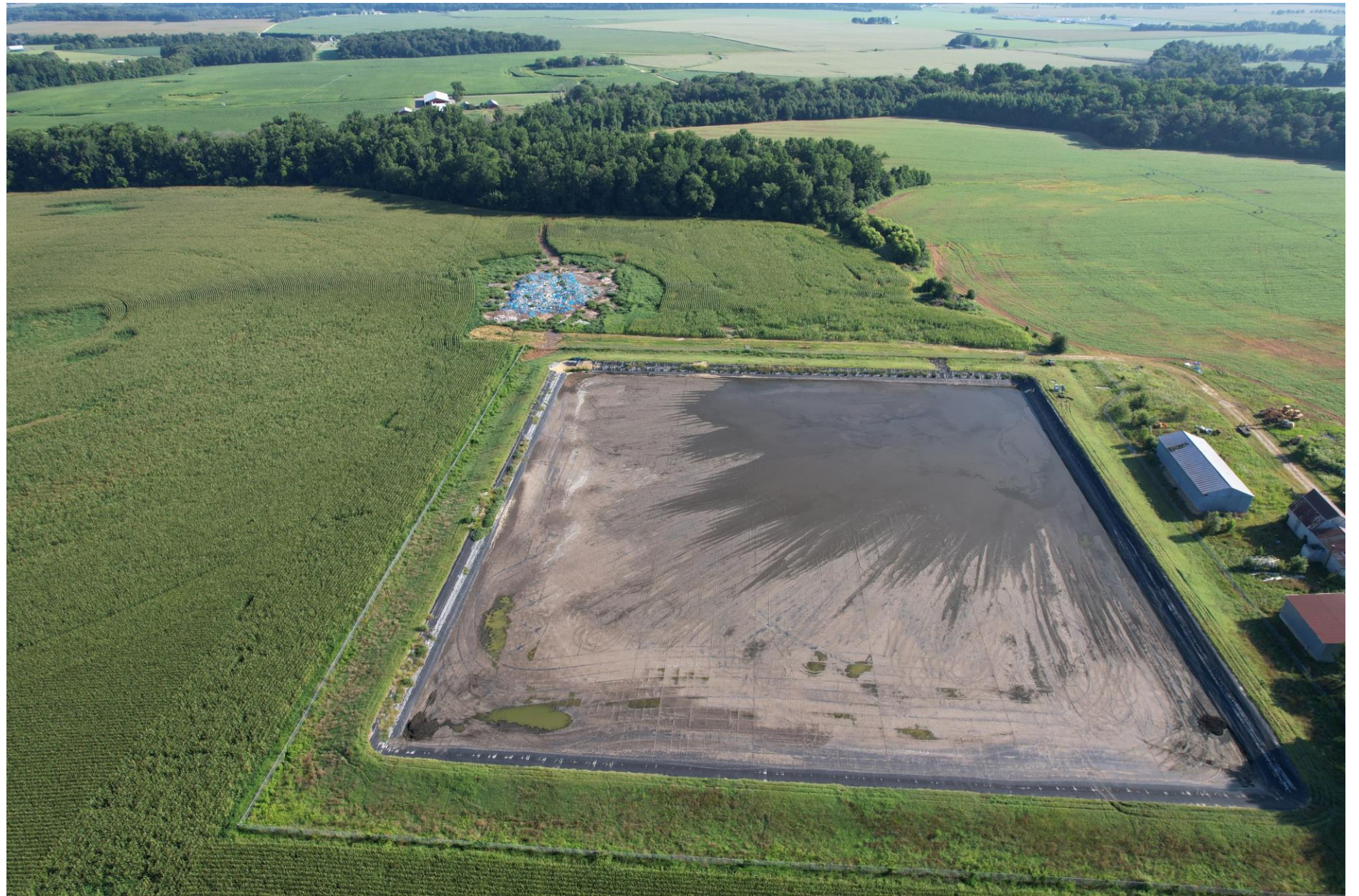
Image 3: Aerial image showing drained wastewater lagoon and solid waste dump (8-14-2023)
