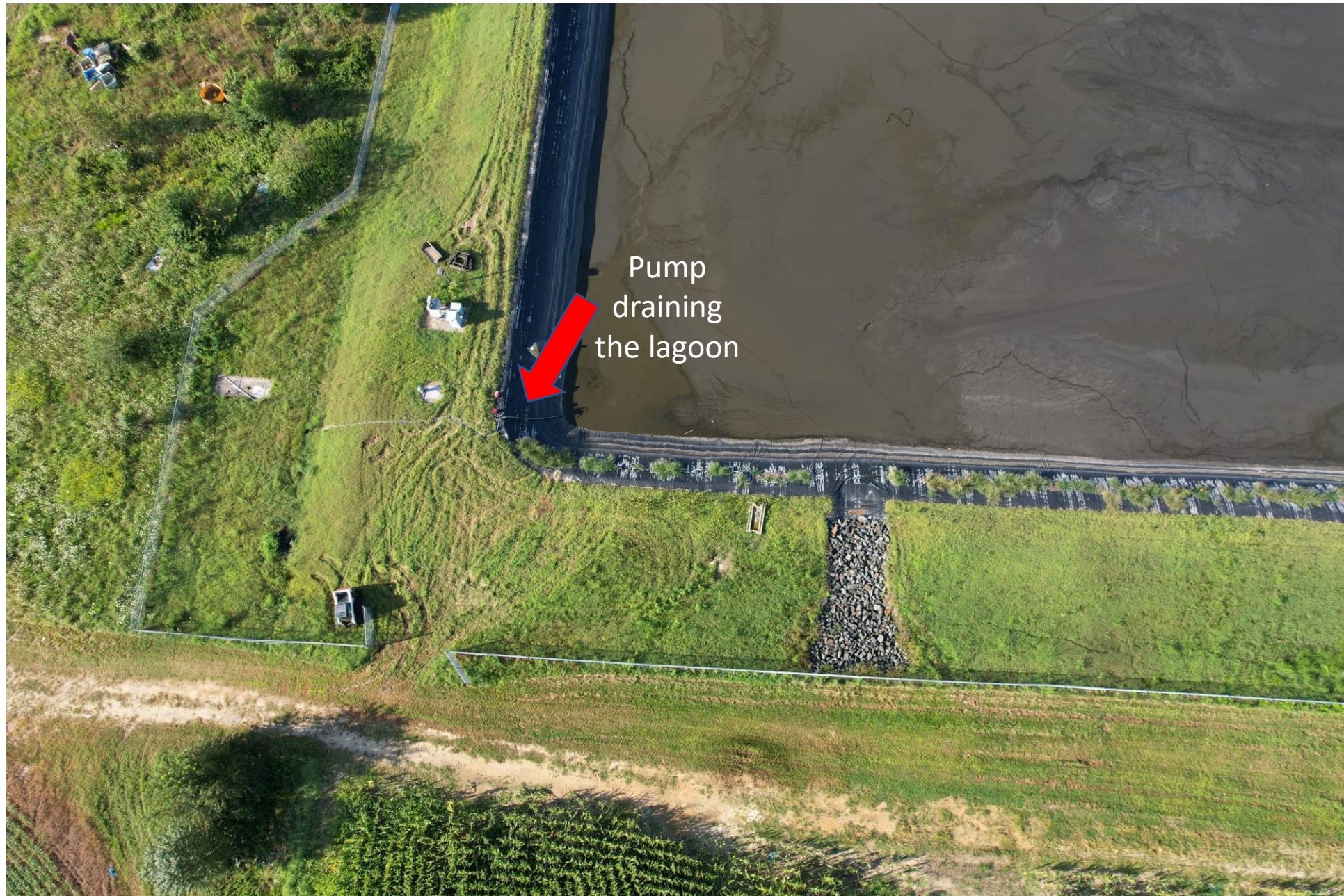
Image 4: Northeast corner of wastewater lagoon showing a pump and hose actively draining the lagoon (8-14-2023)
