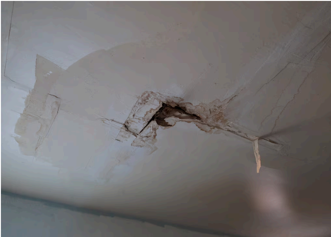
A hole in the roof is causing leaks in Christina Cikins' rental, which she says led to water damage and mold. (KT Kanazawich for The Baltimore Banner)
