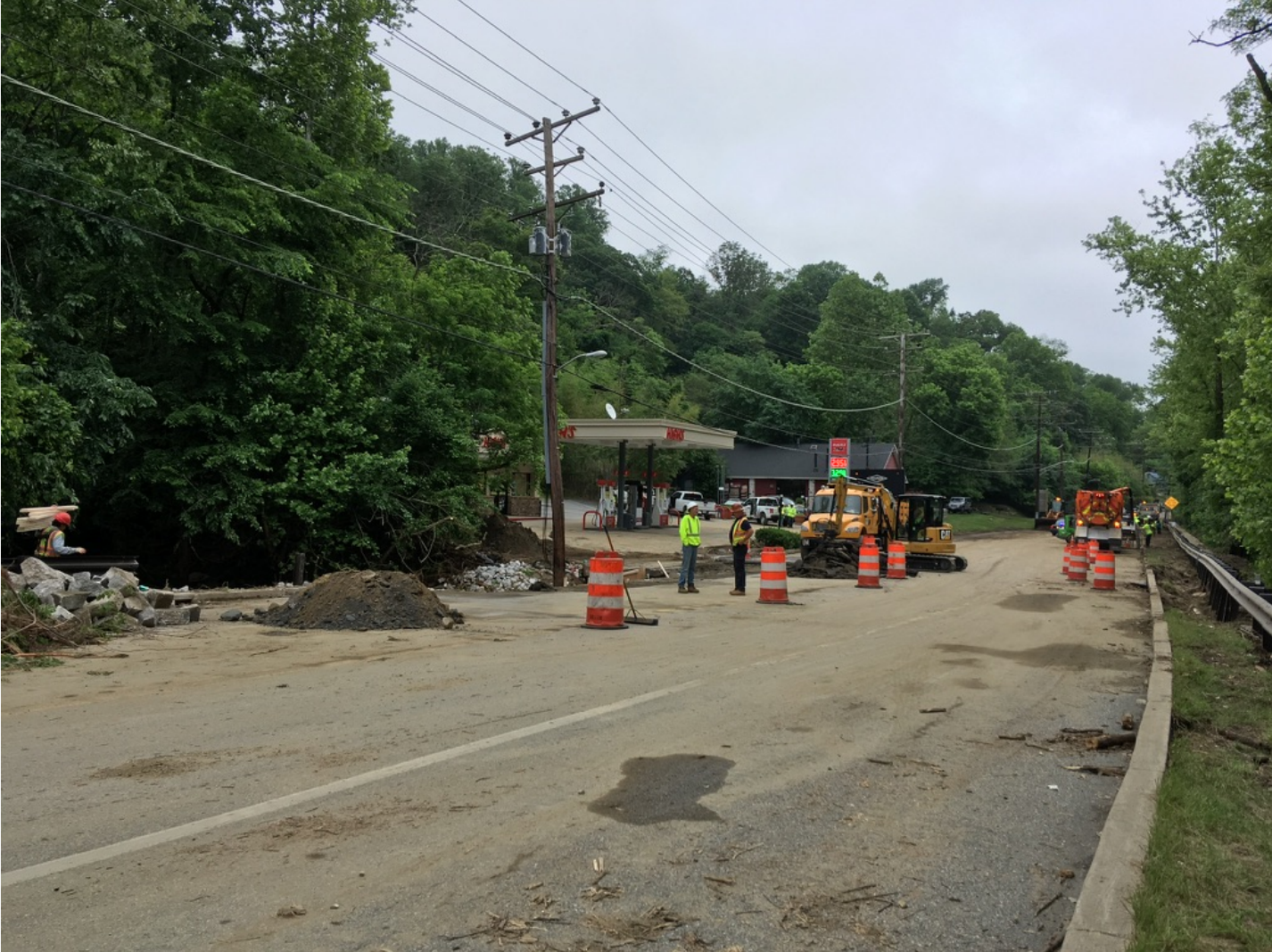
Exhibit 5 Cooper Branch flooding, Frederick Road, Catonsville, 2018
