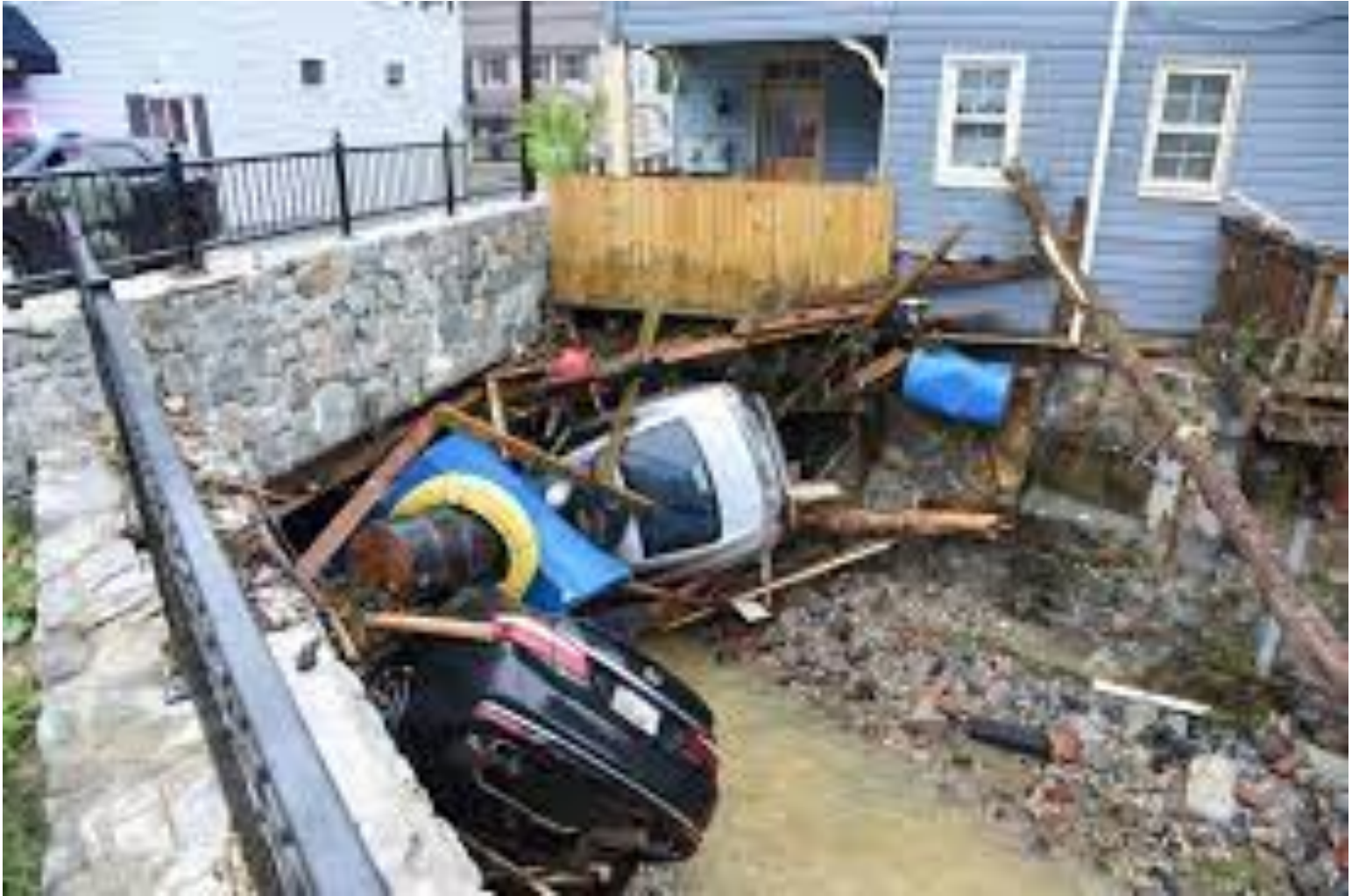
Exhibit two Historic flood damage, Ellicott City. 2016
