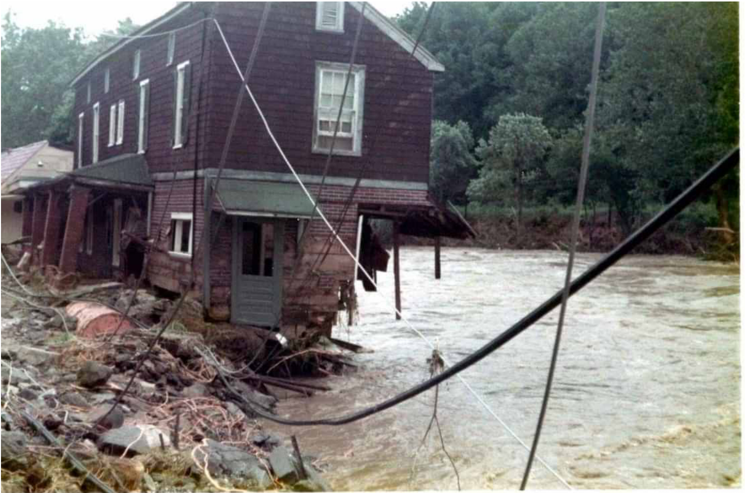
Exhibit four Patapsco River, flooding, Baltimore County 1972
