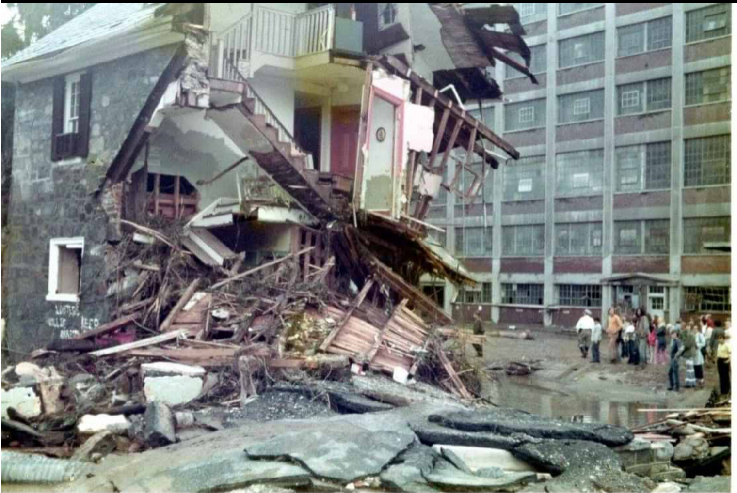
Exhibit three Ellicott Mill flooding, Baltimore County 1972
