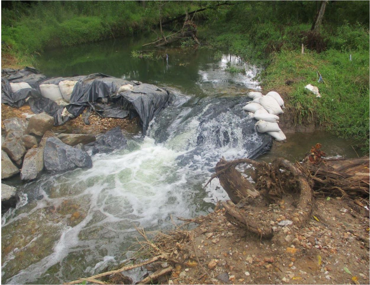
After Stream Restoration Work 2 – Re-engineered streambanks susceptible to blow-outs and heavy erosion.
