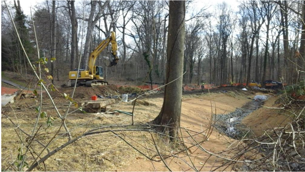
During Stream Restoration Work 3 – Riparian zone cleared of natural vegetation.
