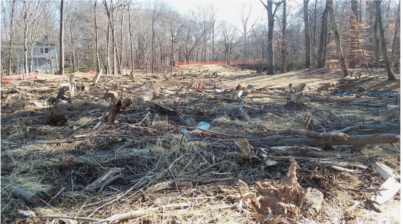
During Stream Restoration Work 1 (Spring 2021) – Heavy tree loss.
