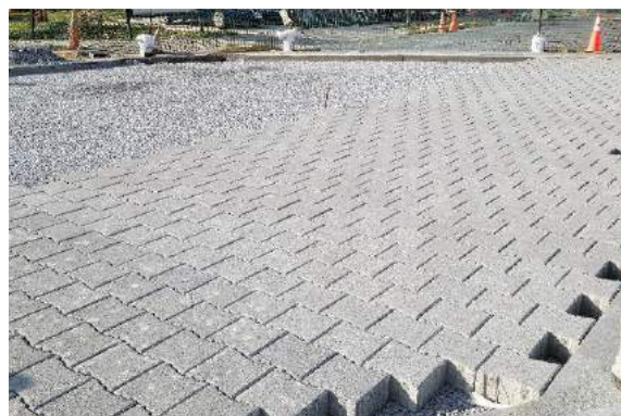
Placement of PaveDrain surface
