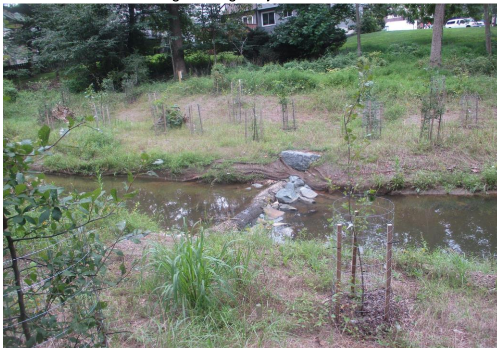
After Stream Restoration 3 – Embankment engineering subject to erosion and failure.
