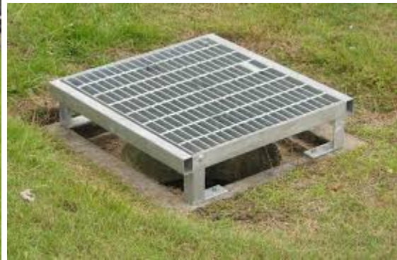
Raised Grate Yard Inlet
