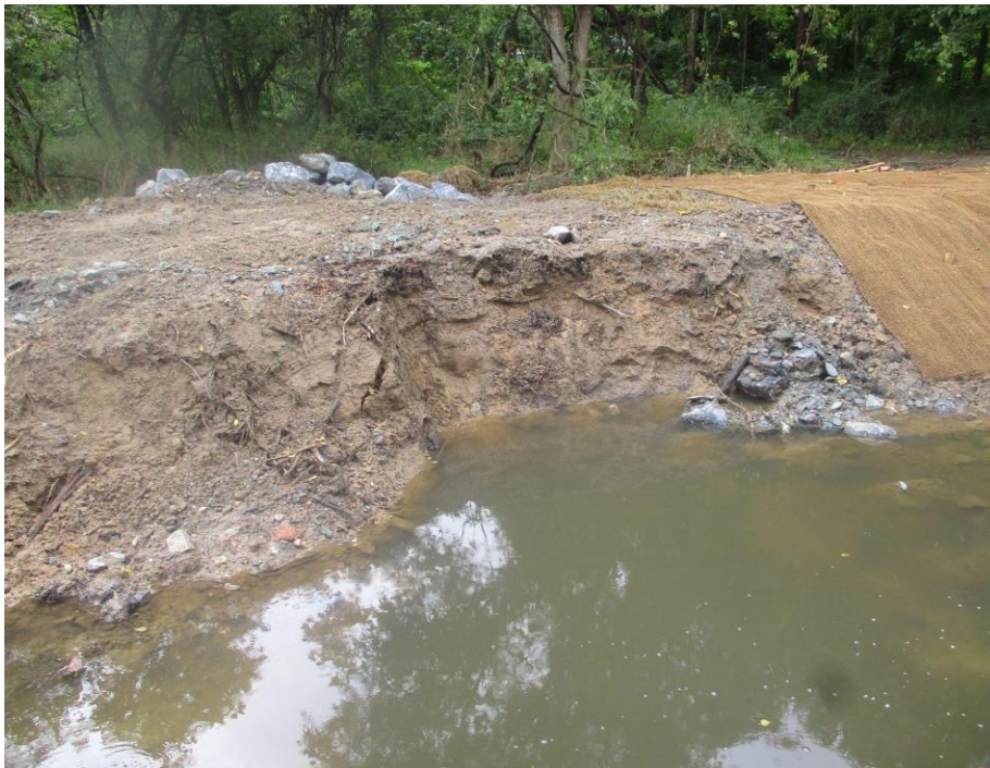
After Stream Restoration Work 3 – Re-engineered streambanks susceptible to blow-outs and heavy erosion.
