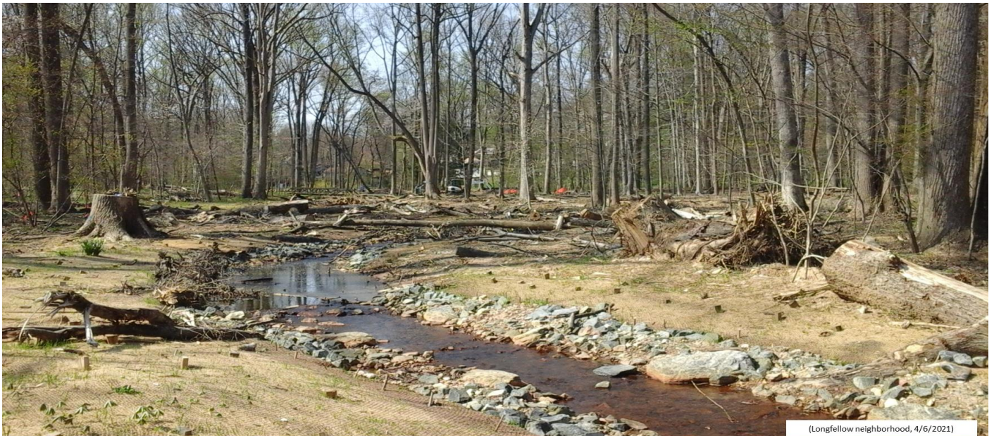
During/After Stream Restoration Work 2 (Spring 2021) – Heavy tree loss, armored stream banks
