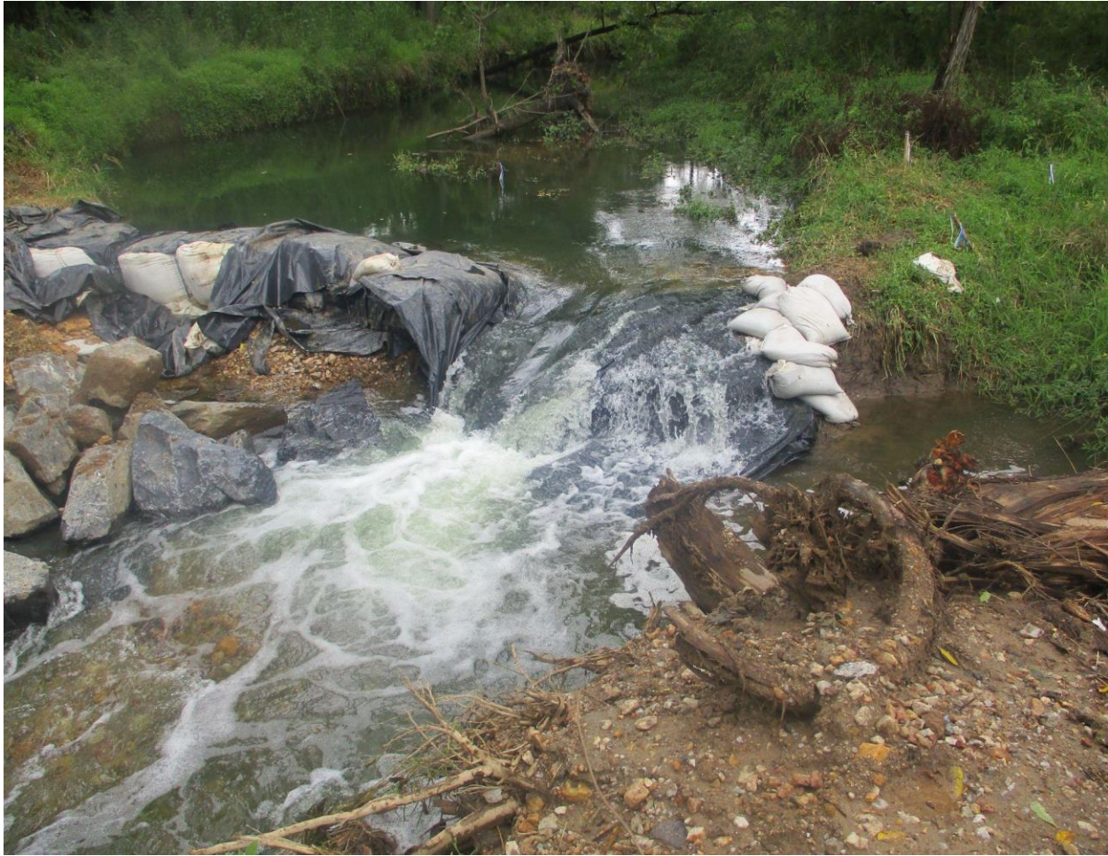
After Stream Restoration Work 2 – Re-engineered streambanks susceptible to blow-outs and heavy erosion.
