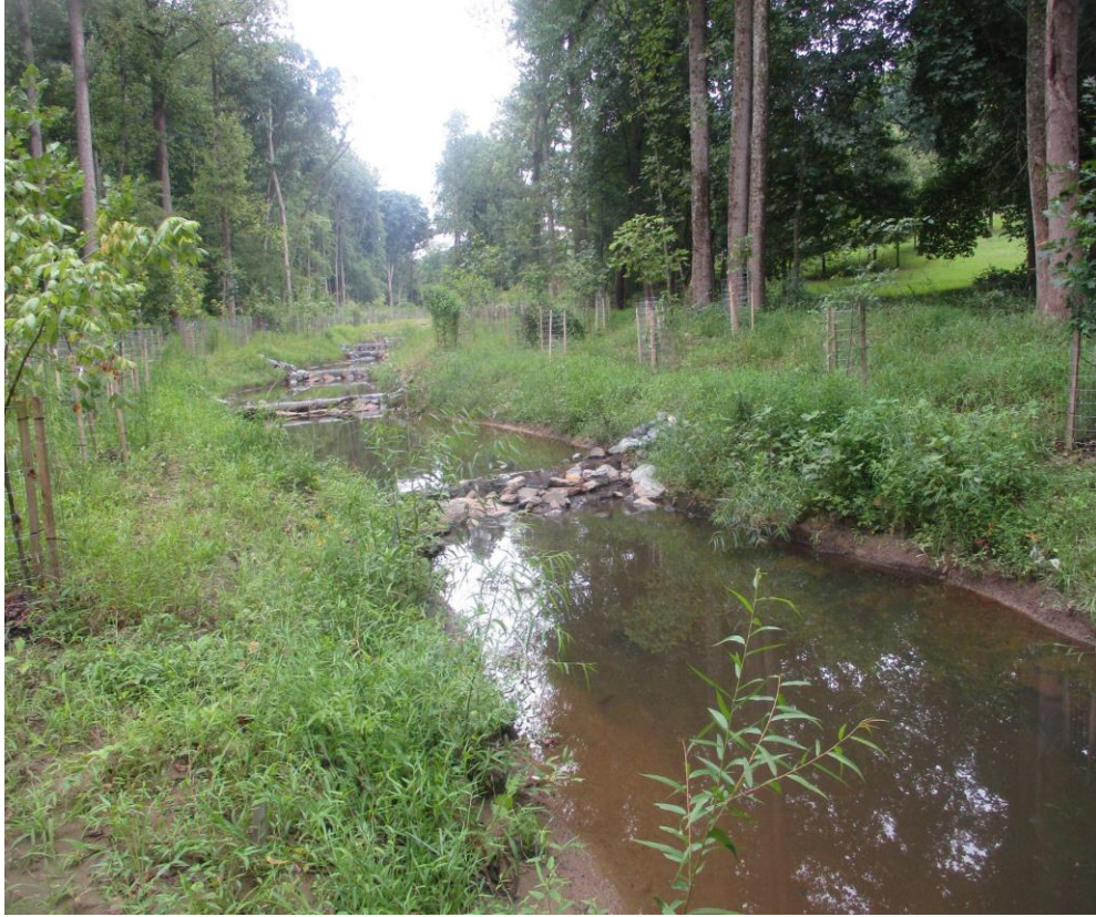
After Stream Restoration 2 – Vegetation dominated by invasive plants.
