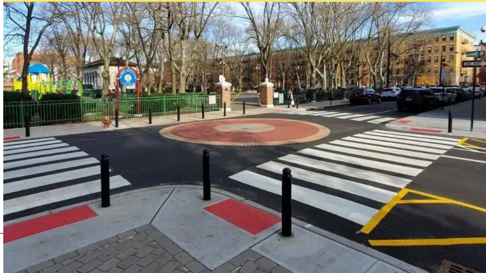
Bottom: A raised intersection and a new crosswalk with wide stripes and reflective paint at Ninth and Grand streets in Hoboken, New Jersey. Photo by City of Hoboken
