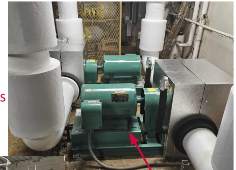
New Chiller Supply Pumps
