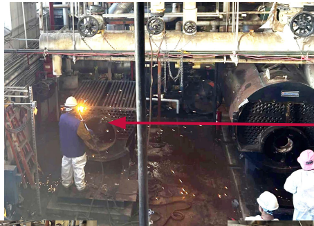
Old Boiler Being Removed
