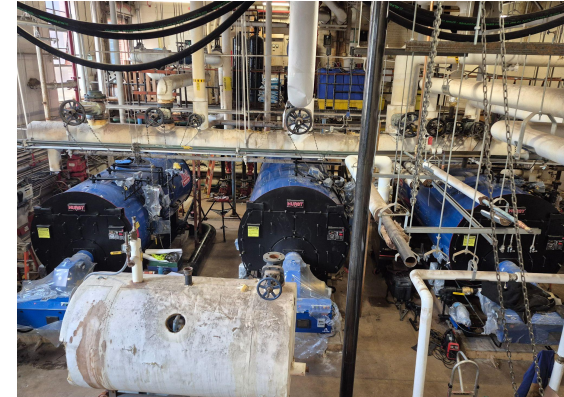
New Boilers Put In Place for Hook Up
