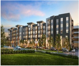
Aspire at Rippon Landing
