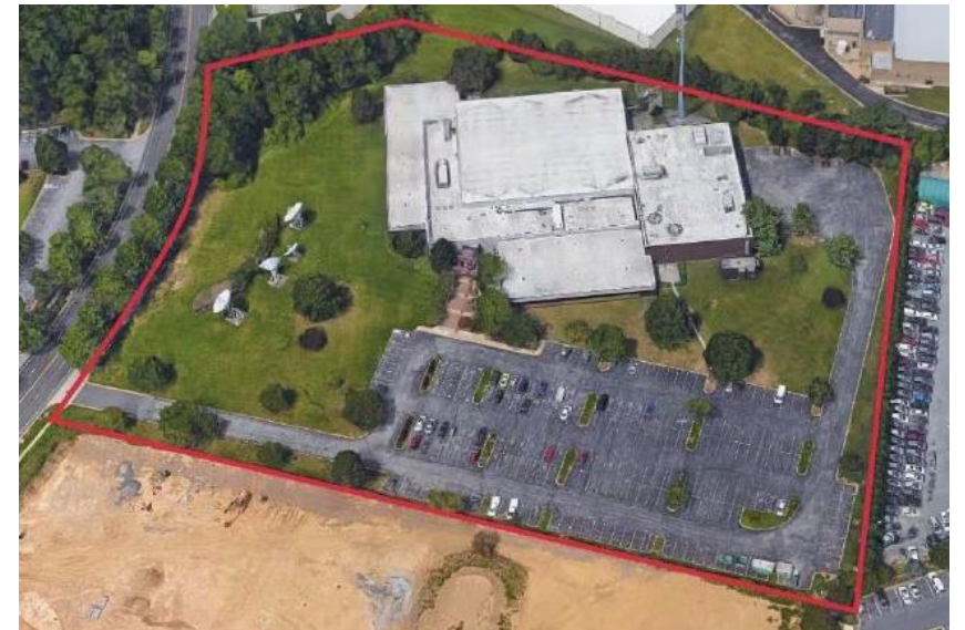
BEFORE: Obsolete Date Center
