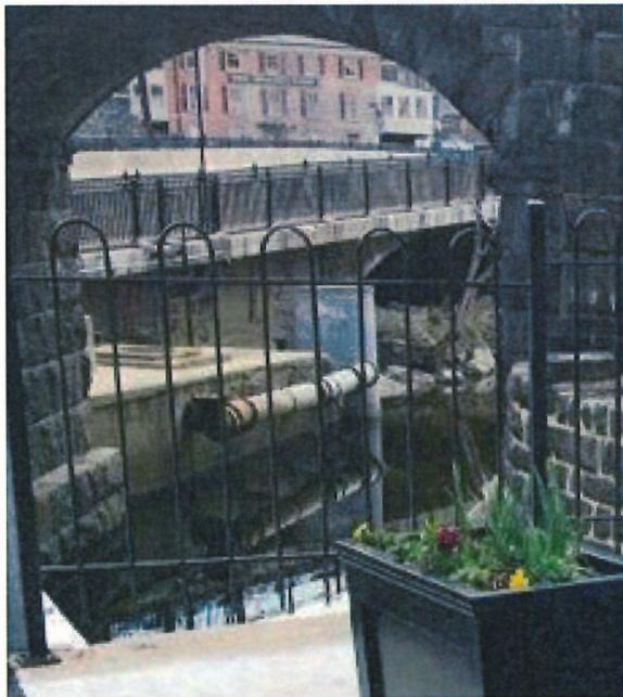
Figure 134: The Oliver Viaduct’s Narrow Opening Restricts Flood Conveyance in Lower Main
