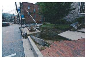
Figure 95: Damage to Brick Paving after the 2018 Flood
