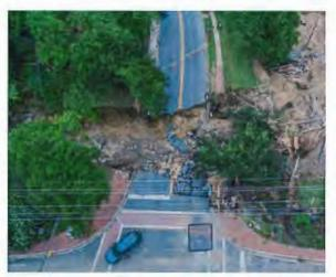
Figure 45: Ellicott Mills Drive Culvert After the 2018 Flood
