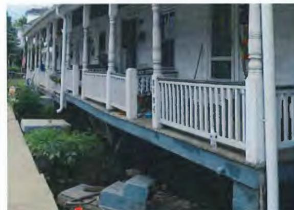
Figure 201: Foundations Scoured by Floodwaters in the West End
