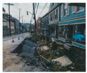
Figure 32: Sidewalk and Utility Damage at 8247 Main Street Immediately Following the 2016 Flood
