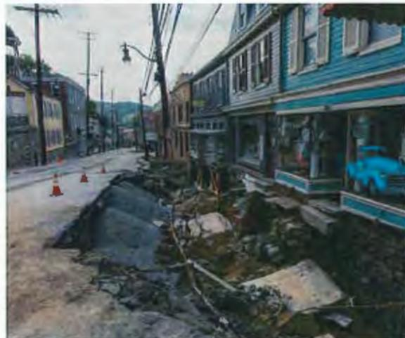
Figure 32: Sidewalk and Utility Damage at 8247 Main Street Immediately Following the 2016 Flood
